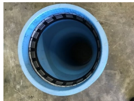
Fully inserted RieberLok Gasket into bell socket with white face marked "Install This Face Out" looking out of the bell.
